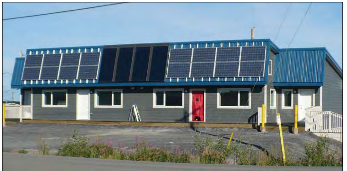
NWTHC photo The Northern Sustainable House in Inuvik.
